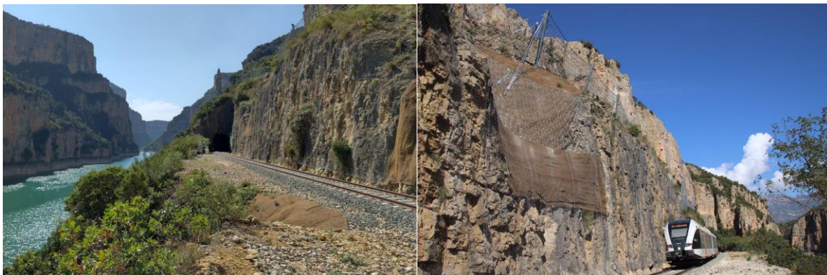
Figure 4: La Pobla railtrack and train circulation under high risk orographic environment
